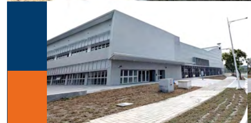
▲ Workshop Building - Aircraft Maintenance Training Center
