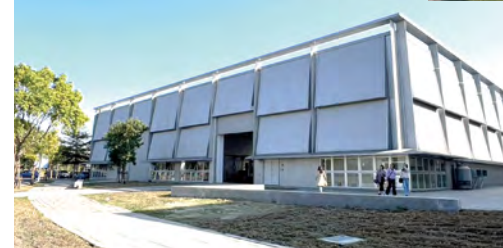
Workshop Buildings 2 and 3 ◀
