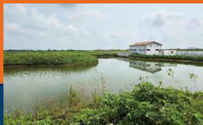
Ecological Retention Pond and Floating Wetland at Full Water Capacity
